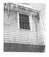
to eliminate the risk by having the ice cleared and installing heating cables to prevent from future build-up. Finally, you may choose to transfer the risk by erecting a barrier and posting signs to warn parents against using the front door; and you may direct them to an alternate entrance. If a parent chooses to ignore the warnings and use the entrance, they are accepting the risk of being harmed; you have transferred that risk to them.
